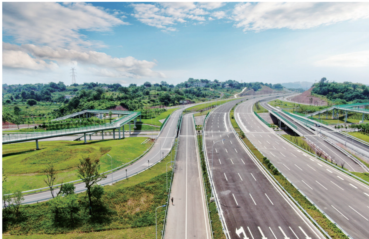
● 泸州二环路(纳溪段)PPP项目蓝安互通立交桥
